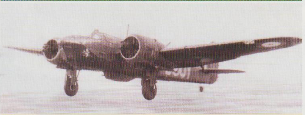
Short flight - V5803 a 254 Squadron Mk.IVF taking off from Dyce on January 30, 1942, only to crash moments later. The elevator trim tab control cables had been reversed and the pilot, Flt Lt Hal Randall was unable to prevent the nose rising the instant it became airborne. Moments later it stalled into the ground, fortunately neither he nor his passenger (the Station Padre!) were injured but a few hasty prayers were uttered.
